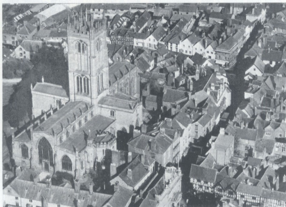
This oblique aerial view of St. Laurence's brings out the huge extent of its roofs and walls, which together give an exposed surface of about one acre.
