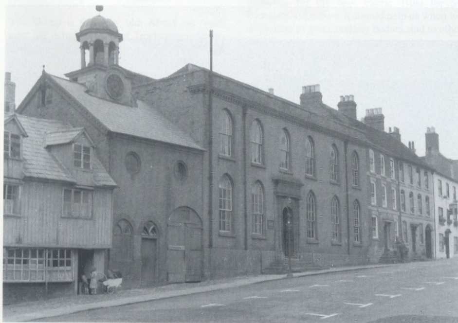
An exterior view of the Guildhall in the 1960s. Though refronted in an imitation Gothic style in 1768, the off-centre position of the entrance is a clue that the interior is much older.
