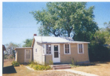
New Ludlow South Dakota, the Old School House
