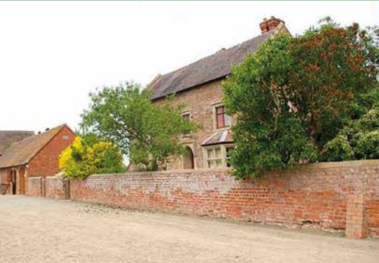
White Abbey Farm in Alberbury. Alberbury priory was founded by Fulk Fitzwarin around 1226 for remission of his sins. The only surviving buildings are incorporated in the farmhouse at White Abbey Farm. They consist of part of the Abbey church and St. Stephen's chapel. FitzWarin and his two wives were buried here. (Image courtesy of https://www.geograph.org.uk/photo/463773 ).
