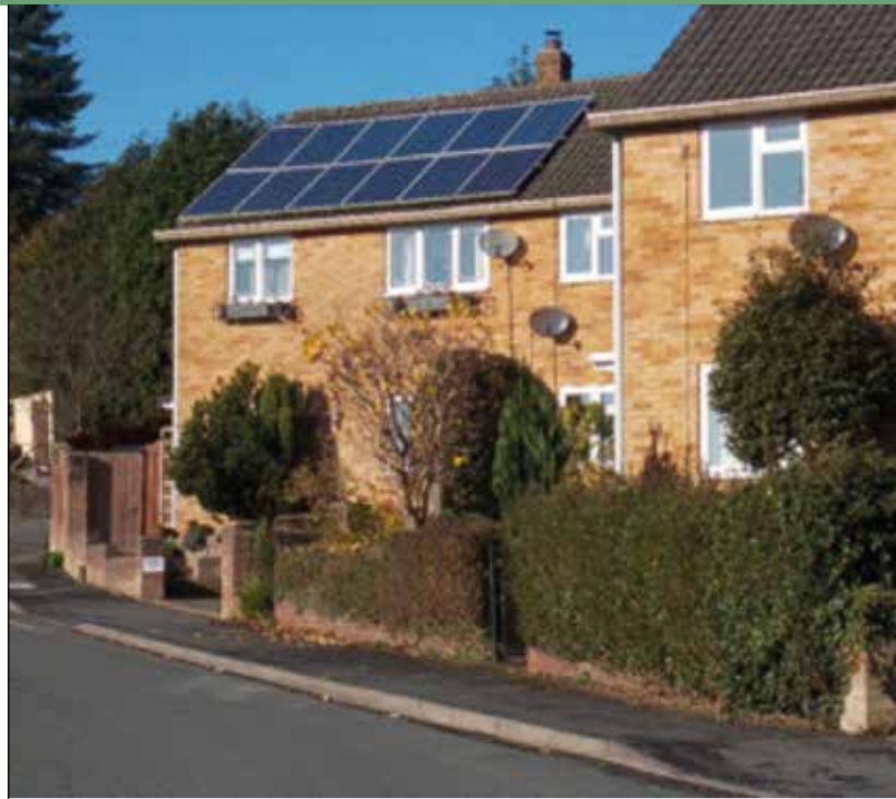
Sidney Road PV panels.
