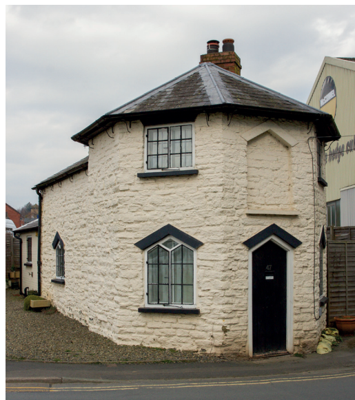
The early 19th century Toll House on the junction between Weeping Cross Road and Temeside.
