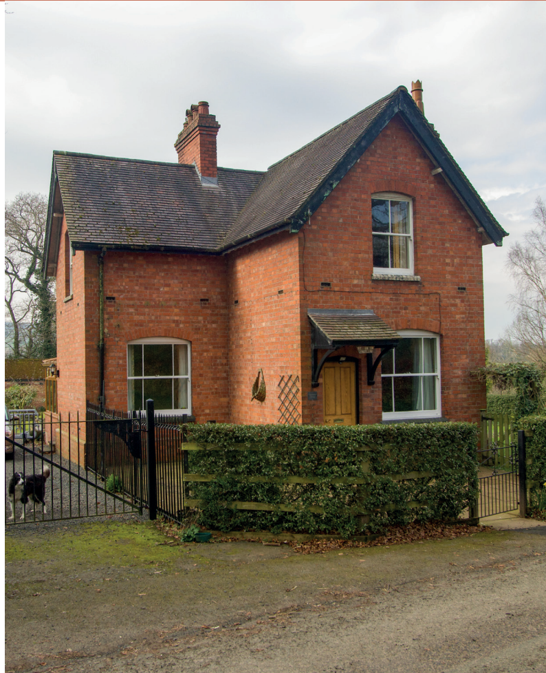
The late Victorian Walkman Cottage – built to house the walkman who monitored and maintained this part of the Elan pipe line.
