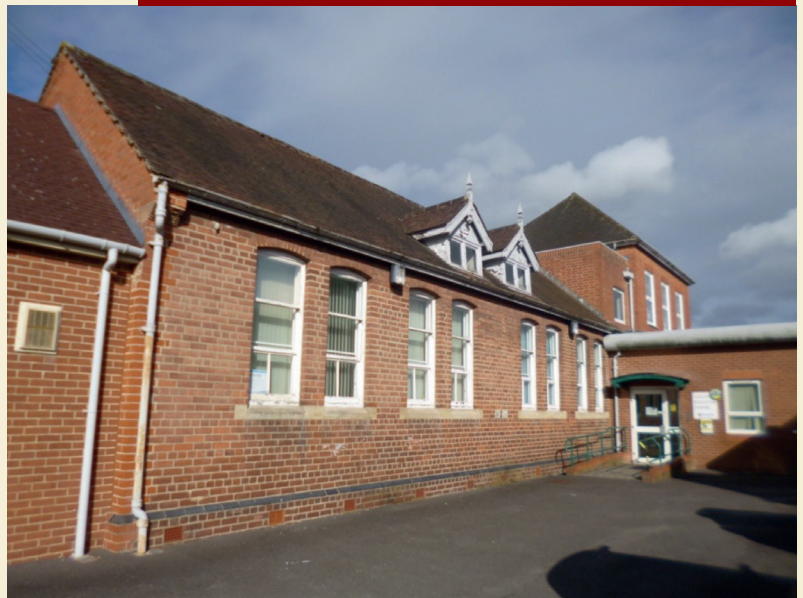
The British School, Old Street. The central part under the two dormers is the original building.
