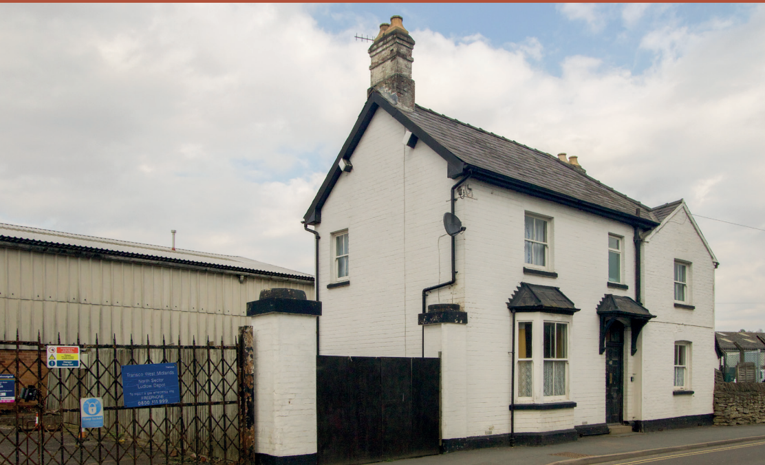
The Victorian house belonging to the manager of the gas works which relocated from Gravel Hill to Temeside in c1840s.
