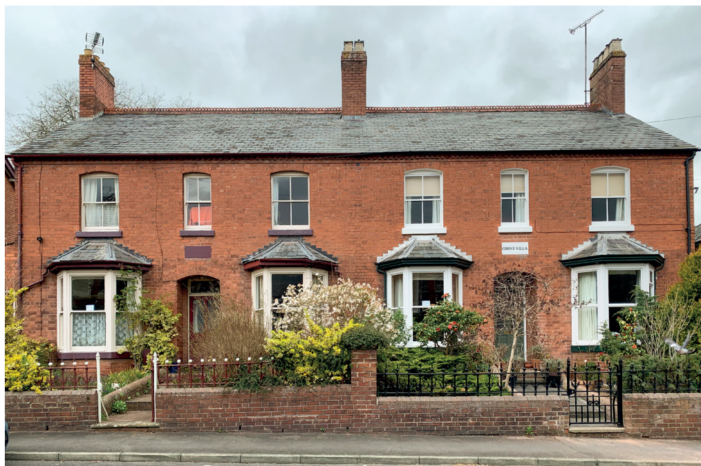
(L) 14 "Park Villa" and 16 "Grove Villa" St. Julian's Avenue.
