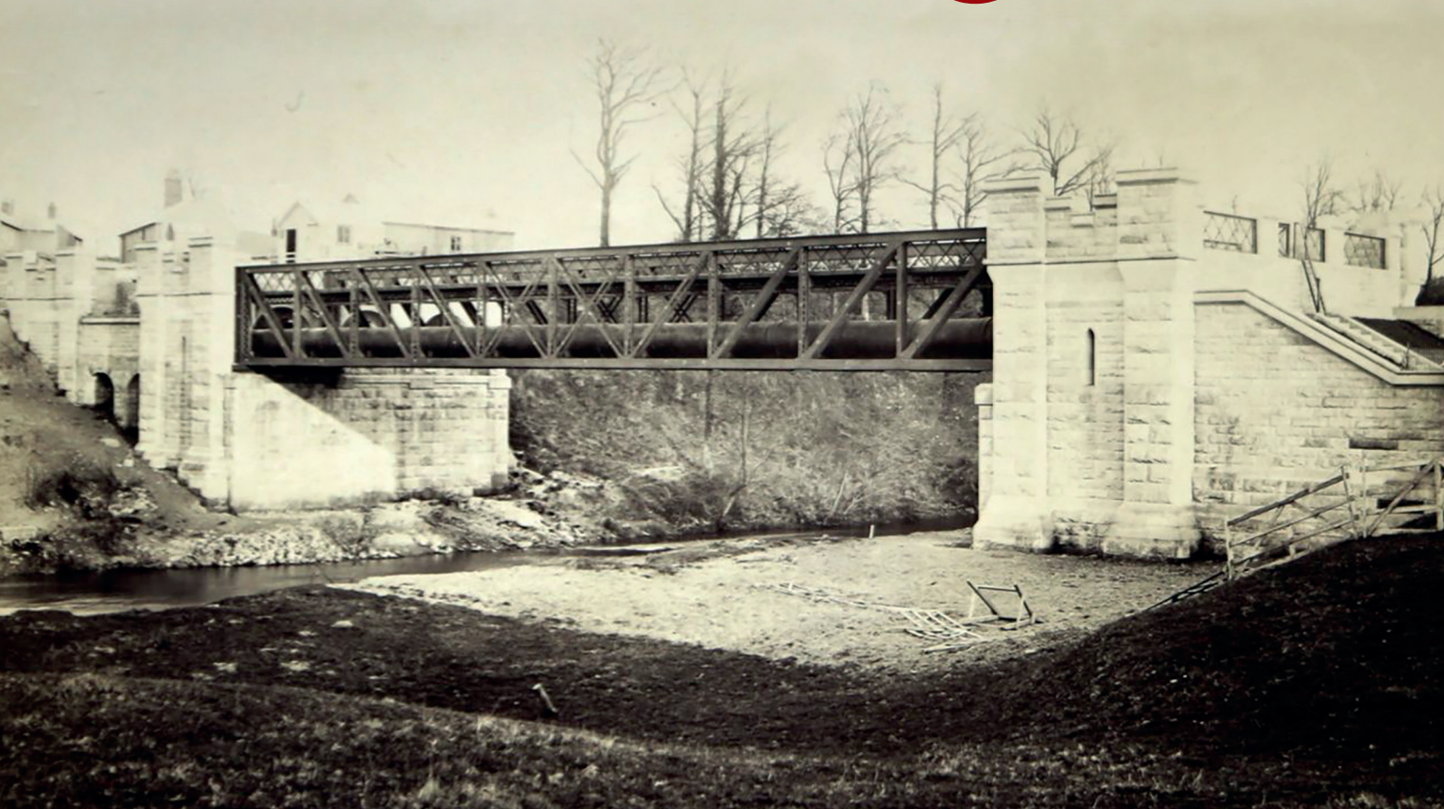
Water-pipe Bridge over Teme at Steventon
