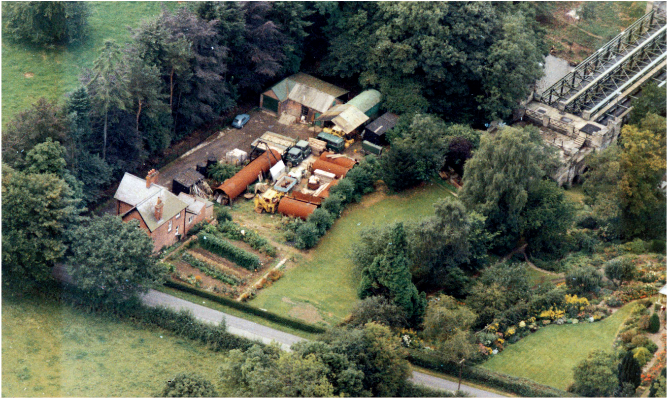
Construction Site at Steventon 1950s
