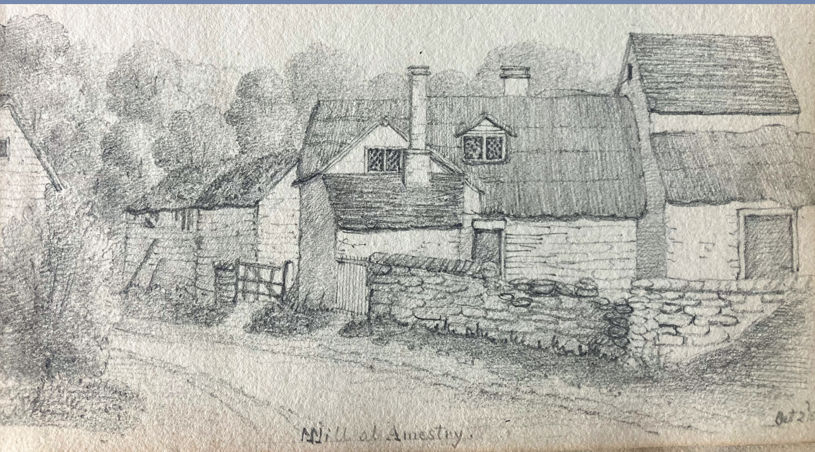
Aymestrey Mill, October 1837, rebuilt following a fire in the 1860s.
