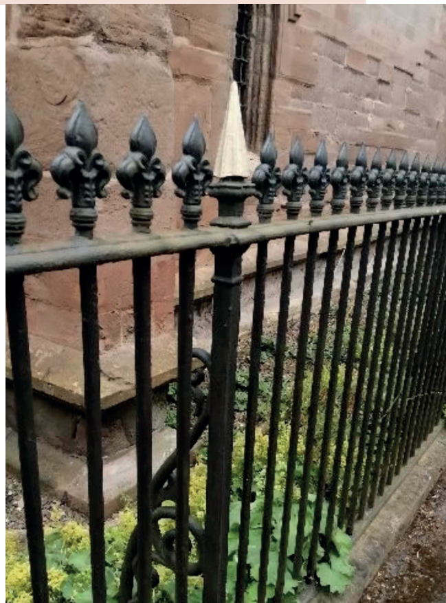
Figure 1. The railings of St Laurence's
